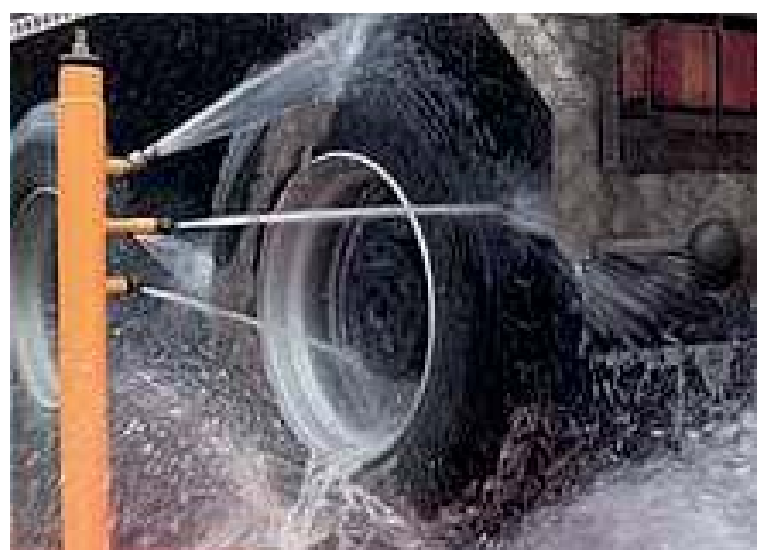
ROAD CLEANLINESS: WHEEL WASH FACILITIES
