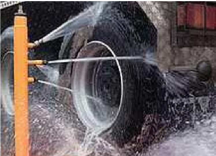
ROAD CLEANLINESS: WHEEL WASH FACILITIES
