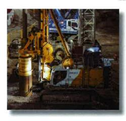
The Piling Rigs have been specially selected following an assessment of the ground conditions as the best equipment for installing the piles with the minimum of disruption.
