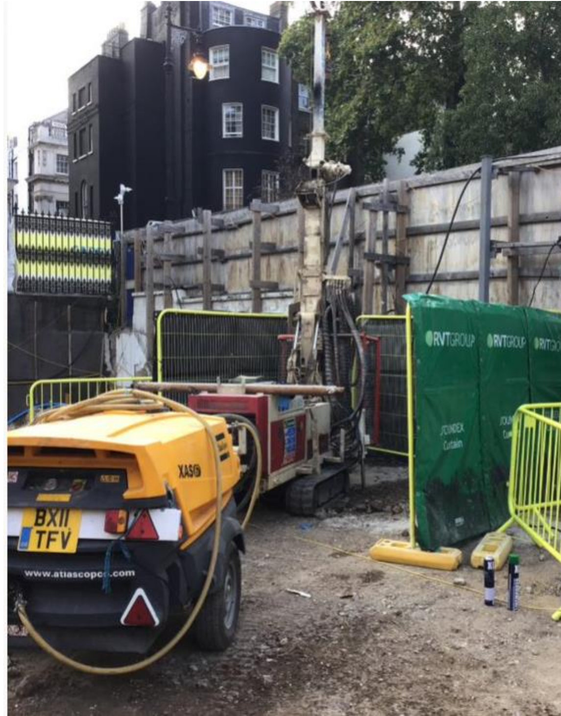
UXO Drilling (With Noise Barriers)
