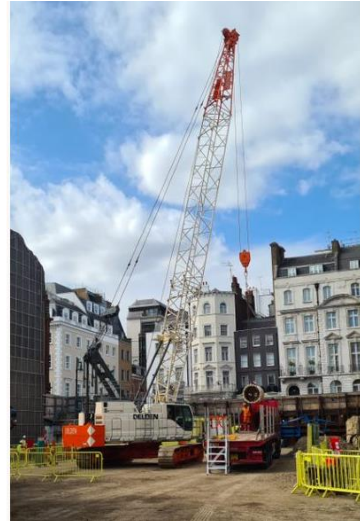
Mobilisation of Crawler Crane
