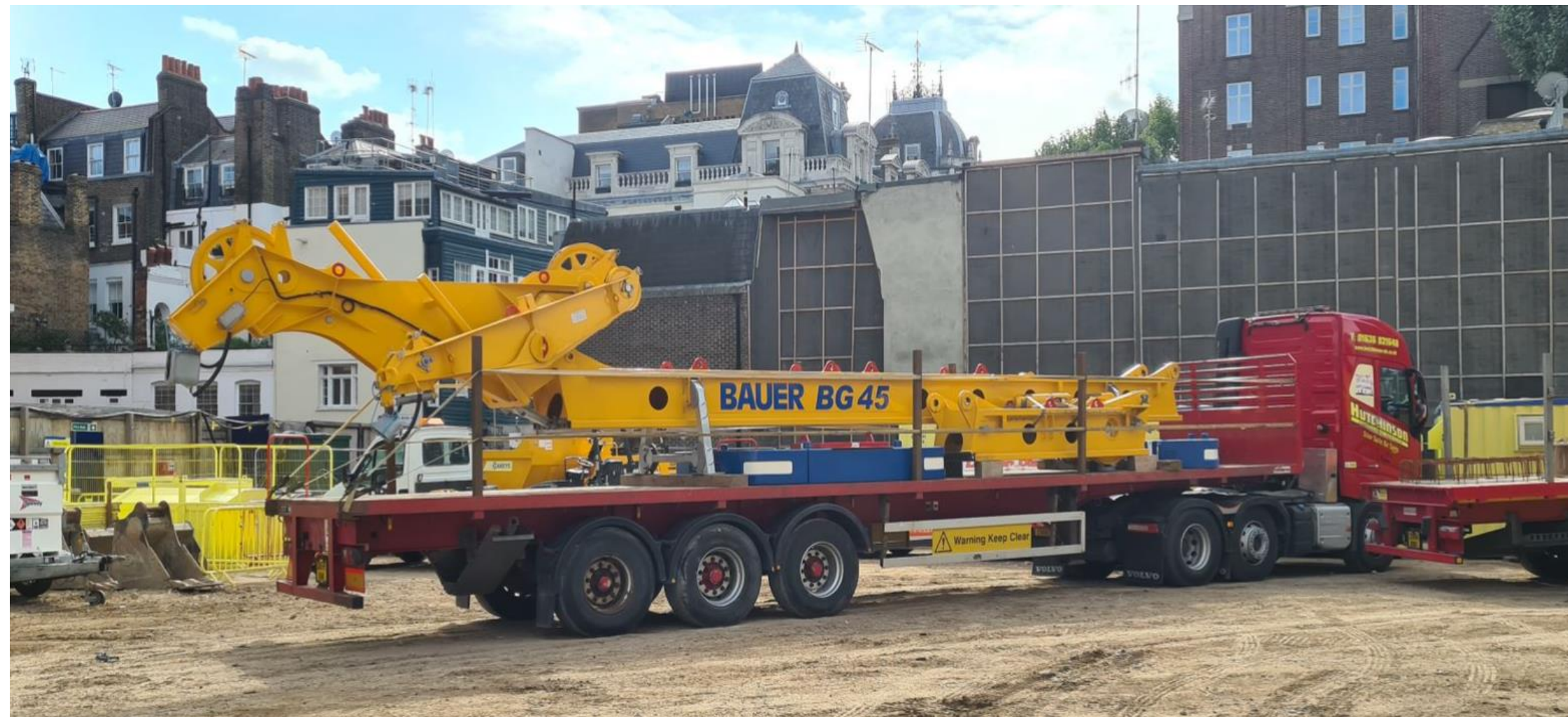
Delivery of Piling Rig Equipment
