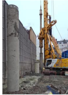
Rig - Installing New Perimeter Secant Piles To South of Site
