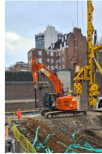
Rig - Installing New Perimeter Secant Piles To South of Site
