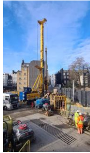
Rig - Installing New Perimeter Bearing Piles To North of Site
