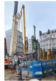
GSHF - Ground Source Heat Pump Mini Rig Drilling
